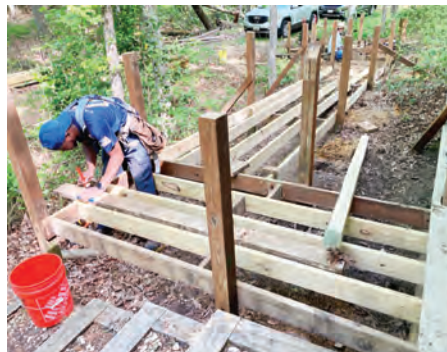
A USA Volunteer works on the boardwalk substructure.
