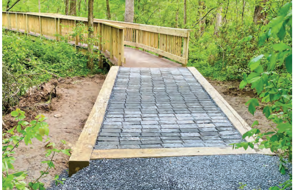
Stone and gravel entryway to the newly completed River Trail boardwalk.
