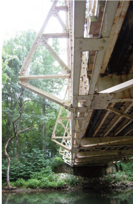
Duvall Bridge before restoration
