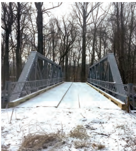
Duvall Bridge after restoration
