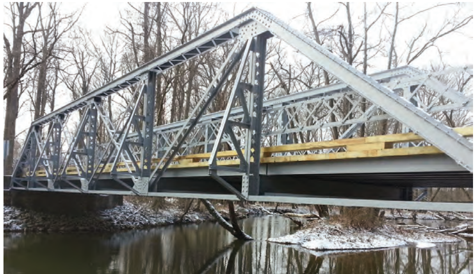
Duvall Bridge after restoration
