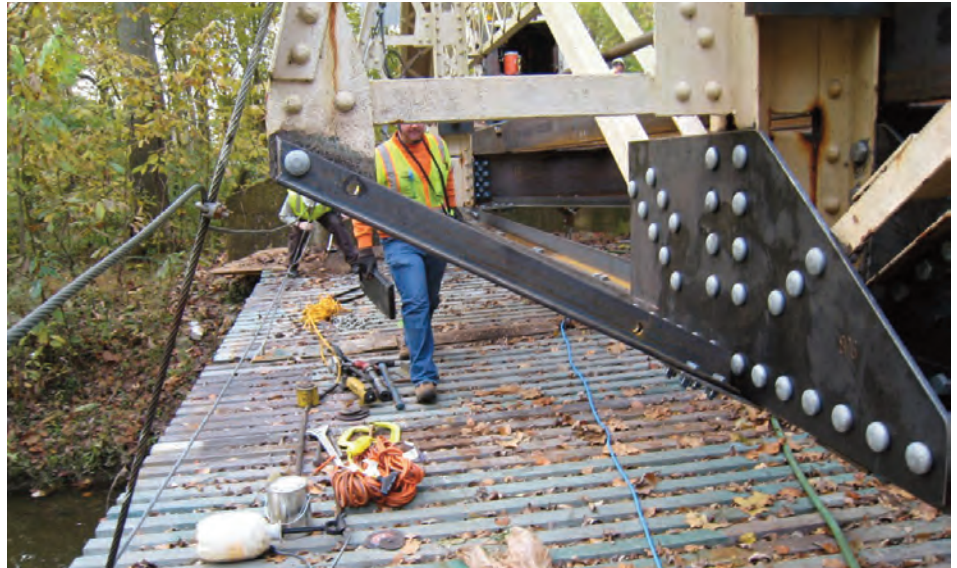
Duvall Bridge during restoration
