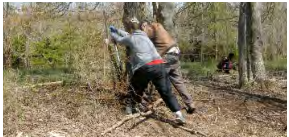
Fence post removal required extra effort.
