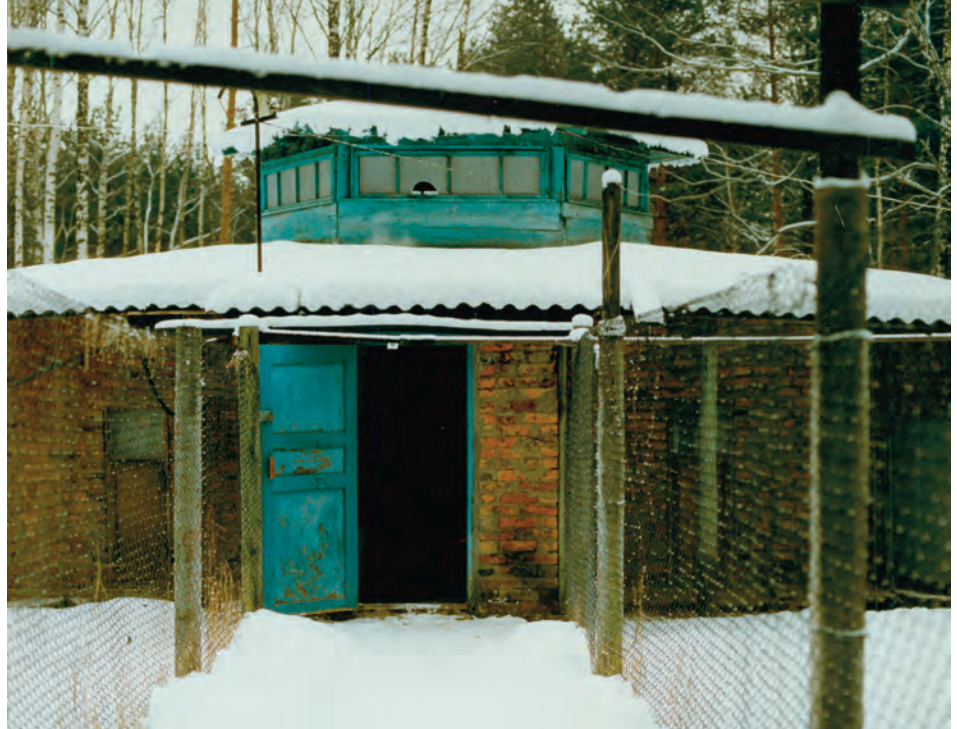
Indoor facility of crane pen complex in Russia
