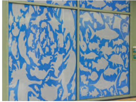
Friend's funds helped pay for the Visitor Center's window treatment to help prevent bird strikes.
