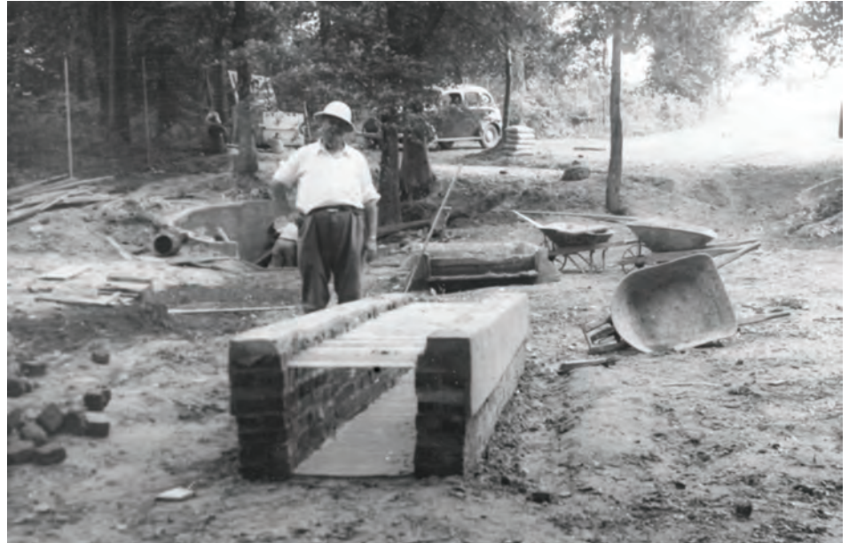
Constructing barbeque pit and spring reservoir for the headquarters picnic ground, mid-1940s.
