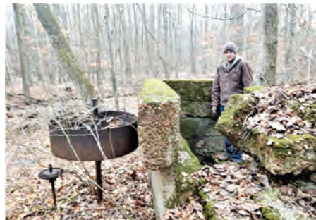
Former Patuxent employee, Oliver Perry, inside old Snowden-Duvall mill structure. On left is the gear and belt wheel above the mechanism (below-ground) that was powered by the water wheel inside the mill.
