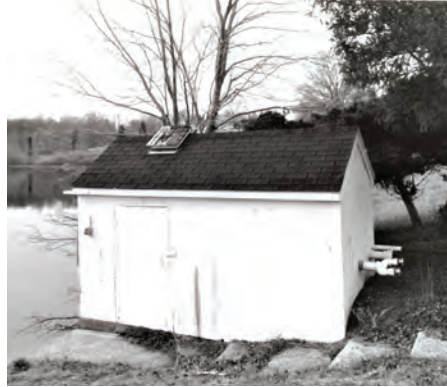
Old Pump House at Snowden Pond.
