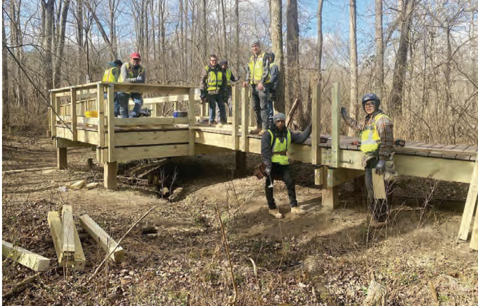
Clark Construction staff working on the River Trail Boardwalk on NT.
